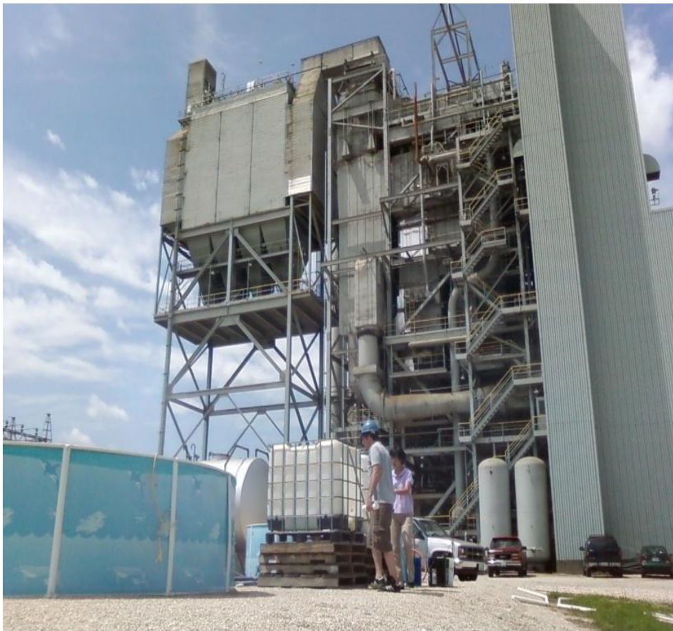
Figure 3.20. Chamois power plant at Central Electric Cooperative at Jefferson City, Missouri.
